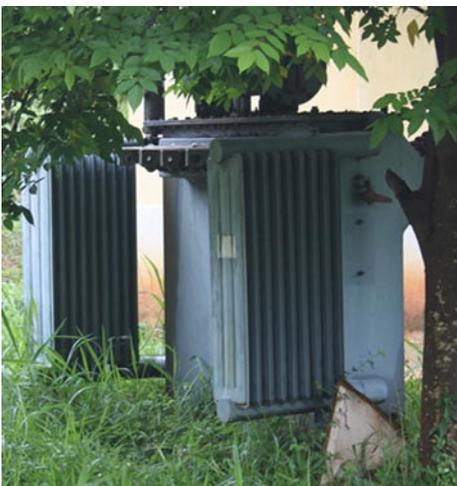
Oil leaking old transformer
